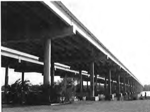
Figure 4.7 – Arrow-S Boat Launch under IH 820
