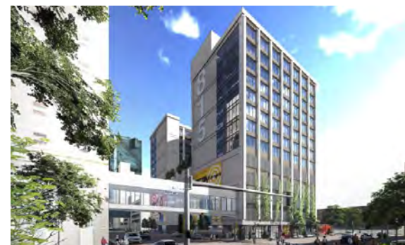
The DDRB approved renovation plans for the 13-story Hotel Texas Annex on Commerce St. The hotel could open early 2023.
