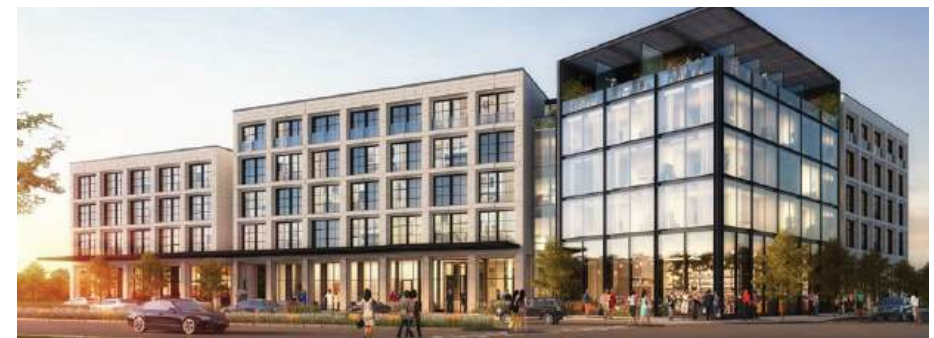
Location: Proposed Crescent Hotel, 3300 Camp Bowie Boulevard
