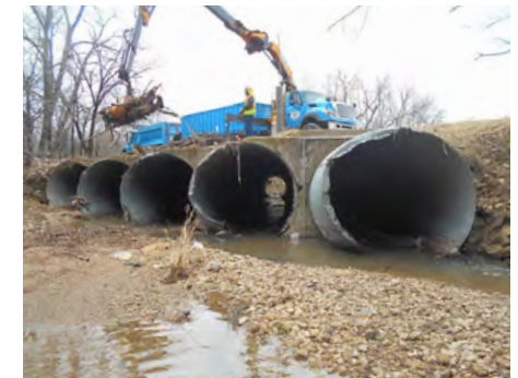
Clearing debris from storm drains.
