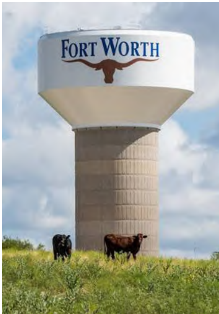
One million gallon elevated water storage tank in Parker County, constructed north of I-20 to serve development in far west Fort Worth.
