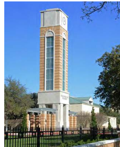
The Texas Wesleyan Bell Tower was constructed as part of a new Texas Wesleyan University main entrance. The new entrance, together with the East Rosedale Renaissance streetscape improvements, enhance student safety and effectively connect the University to the East Rosedale Street store fronts. (Source: City of Fort Worth, 2016.)
