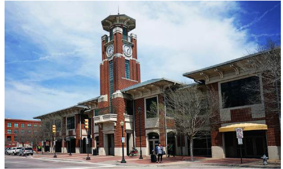
The Fort Worth Central Station, at the intersection of 9th Street and Jones Street in Downtown Fort Worth, exemplifies the value that Fort Worth assigns to mobility. This facility, which opened in January 2002, serves as a terminal for seven transportation modes, including commuter rail services between Fort Worth, Dallas, and the Dallas Fort Worth International Airport. (Source: We Are Dallas Fort Worth Blog, wearedallasfortworth.com )
