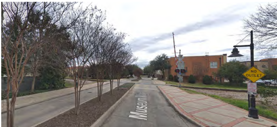
Example of an enhanced crossing in a quiet zone on Museum Way. In order to prevent drivers from deliberately driving around lowered railroad gates in this quiet zone, a median barrier is placed in the center of the roadway.
